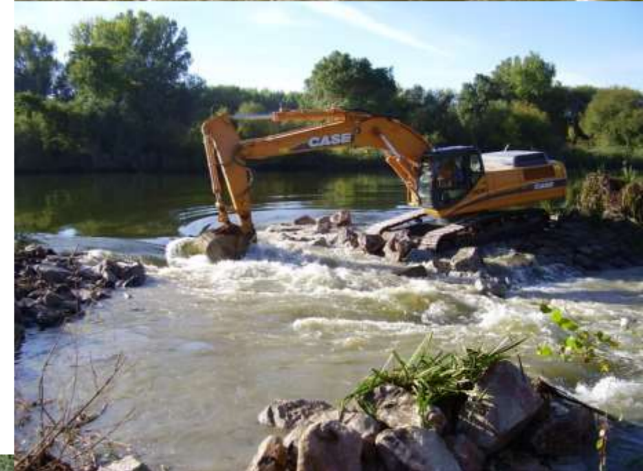
Demolition of La Concepción weir (Tormes river, Salamanca-Spain)
